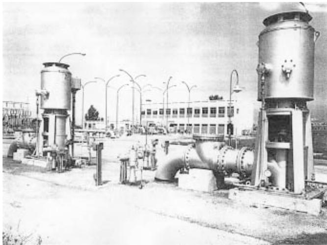
Fig. 3: Pumps with measuring transmitters in the field with an operating building in Ingolstadt
